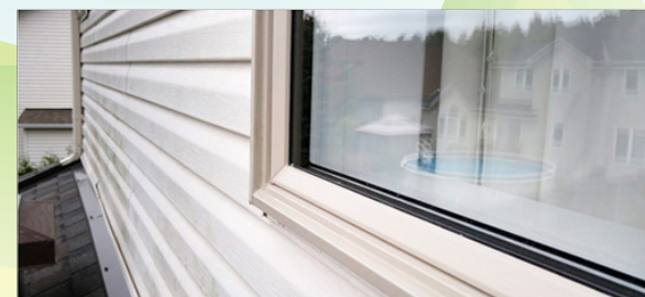
No sash - Exterior
